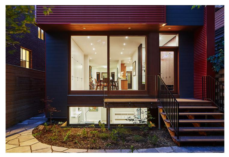
At the back of the house, the architects added a new, two-storey volume clad in red corrugated steel.
